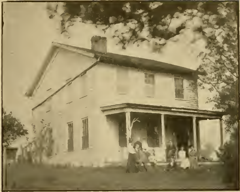
THE OLD GORDON HOMESTEAD, 7th Street.
